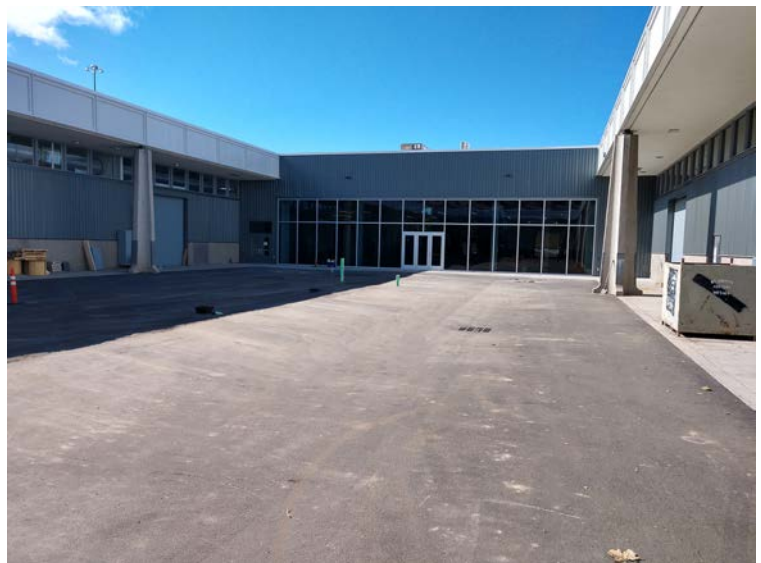
Courtyard area, still under construction
